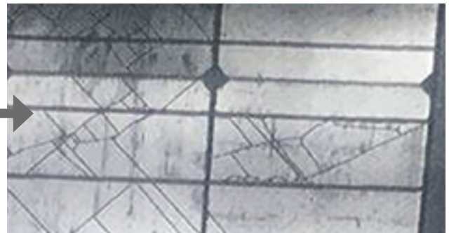
Micro-cracks detected (EL imaging)
